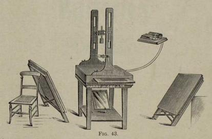
The skin-window can be placed in the middle, or at either end of the couch. It is supplied with a mirror to enable the operator to see upon the screen that portion of the body which he is engaged in radiographing. And the Tube can be placed either above or below the patient, as desired.
