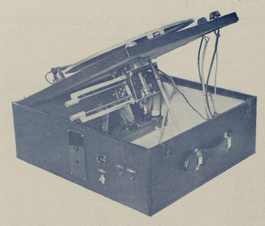
This unit will at once appeal to commercial users, and enthusiasts. The general specification is as the S.T.R. unit, with the addition of the amplifier, which is specially matched to the D.T. 7 recording head, and is adjustable for 200, 220, 240 A/C mains. All the wiring is carried out inside the case and volume and tone controls are on top of the motor board.
